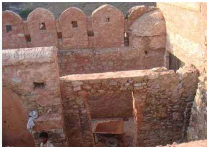
Figure 1-3. View of excavated tunnel from Amber Fort to Jaigarh Fort which housed the gunfoundry of Kachchwaha Rajput Kingdom, Rajasthan (Image by Shikha Jain)
