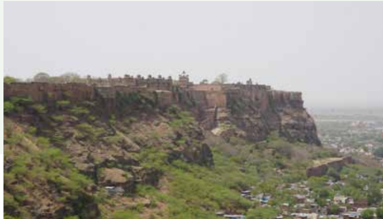
Figure 1-4. Gwalior Fort, Malwa Sultanate with 16th and 17th century structures from Mughal period (Image by Shikha Jain)
