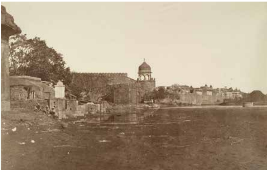
Figure 1-1. Water Gate of Red Fort, Delhi, 1868 ( Source: Archaeological Survey of India)
